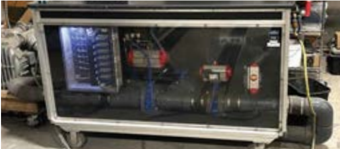
Structural Control Panel
